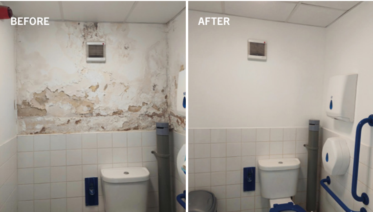
Water damage caused by the roof leaks
